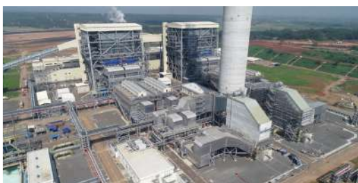
Stack: Boiler Backend Area
