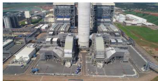
Absorber Unit #1 & Unit#2
