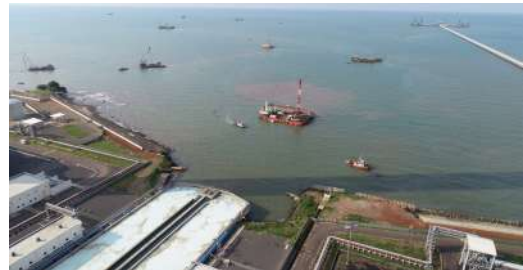
CW Pipe OUTFALL Line
