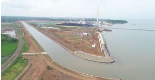
Storm Water Discharge Channel
