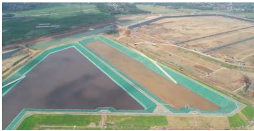
Ash Yard Sedimentation Pond
