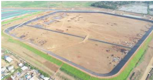
Solid Waste Disposal
