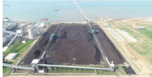
Coal Yard Area
